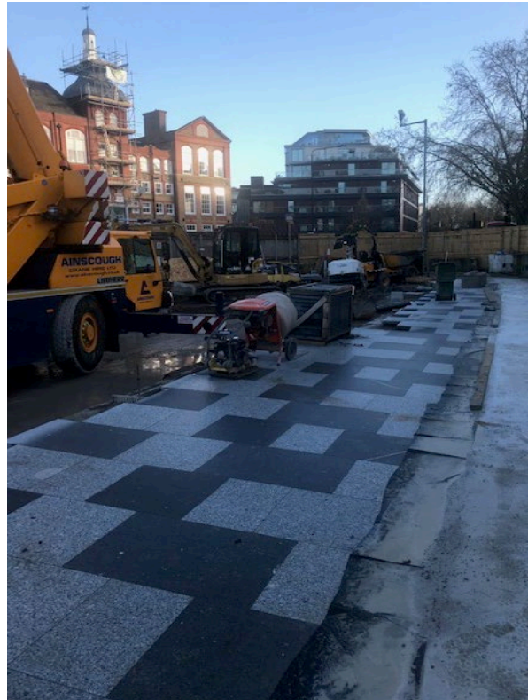
Figure 4 - New granite paving at the Green
